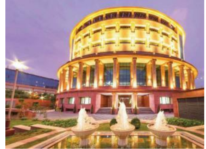
State of The Art Building - Office Complex for Supreme Court of India - Delhi
