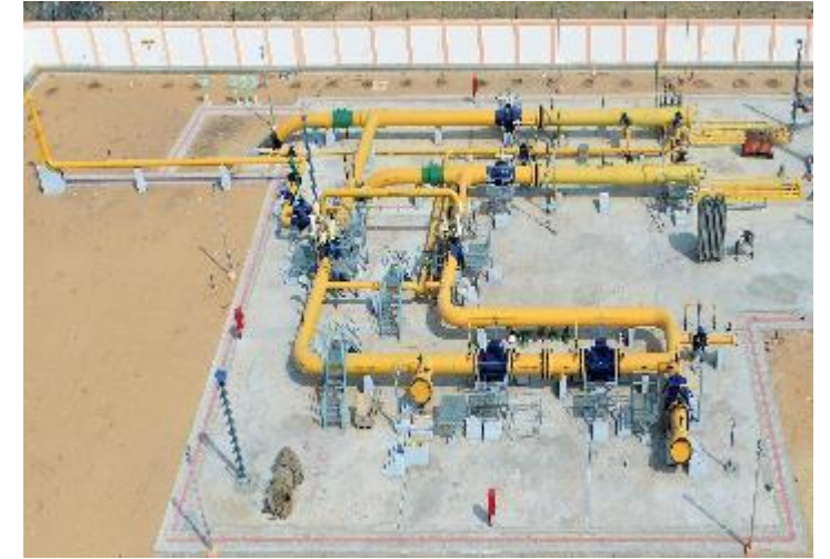
Mehsana Bathinda Pipeline Project Spread IV – GIGL - Rajasthan
