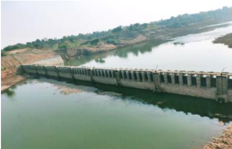
30 MLD at Khargone & 50 MLD at Burhanpur, Urban Water Supply Schemes, Madhya Pradesh
