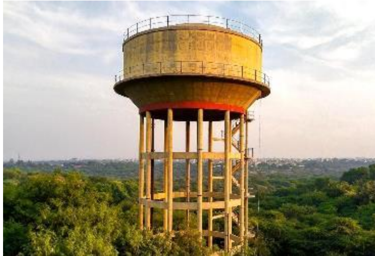
Break Pressure Tank and MS Pipe Gravity main | 360 MLD of water | Length - 39 kms, Madhya Pradesh
