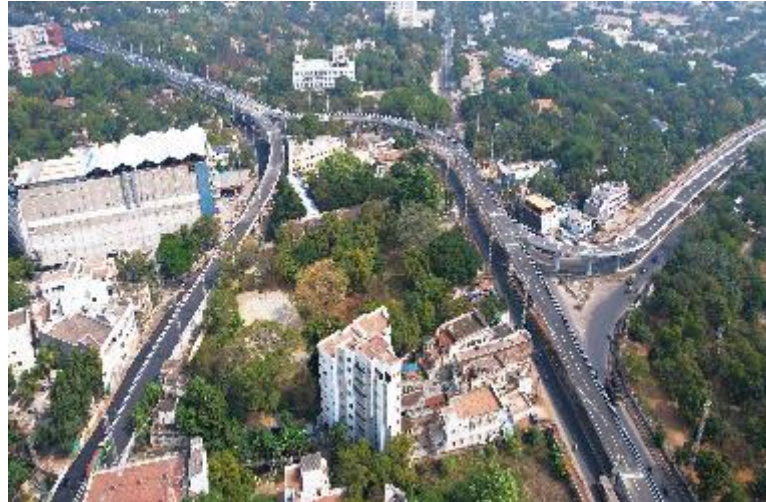
Four Laning of Madurai - Chettikulam - 7.3 km
