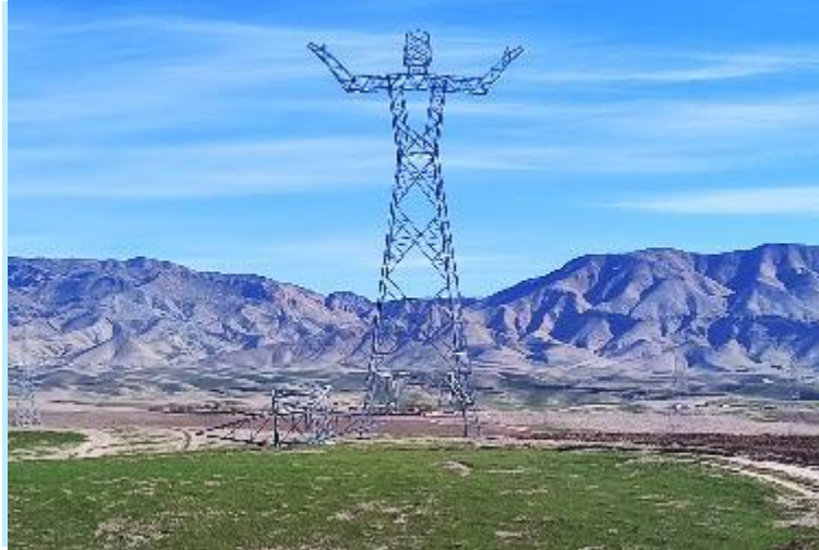
500 kV HVDC 200 Km Transmission Line from Tajikistan Border to Afghanistan
