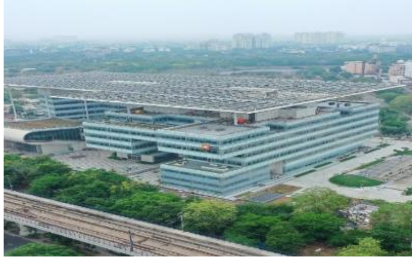
Rural Electrification Corporation World Headquarter Building, Gurgaon, Haryana.
