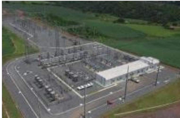
Substation works in Brazil
