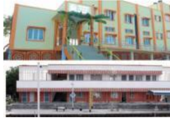
Madurai Tuticorin Doubling Project
