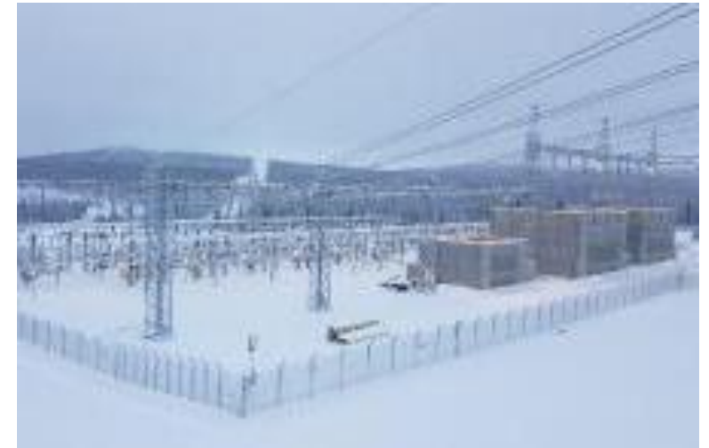
Substation works in Sweden
