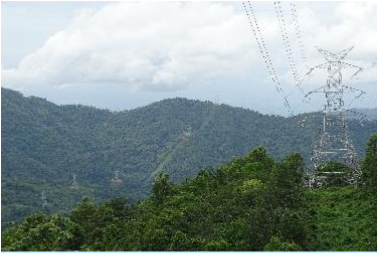
500 kV D/C 167 Km Transmission Line in Thailand
