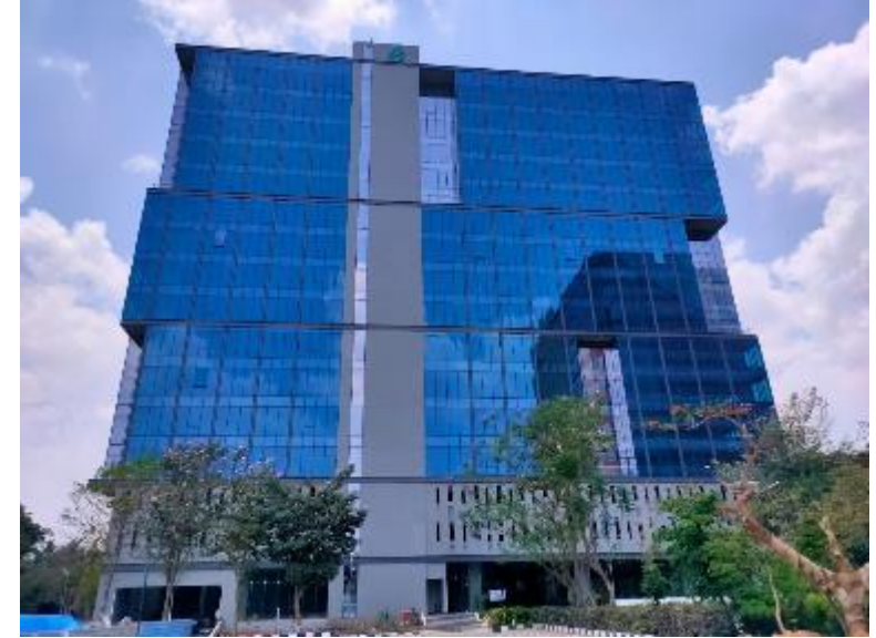
Development of Multi Tenanted Building (MTB5) – ASCENDAS, Bengaluru
