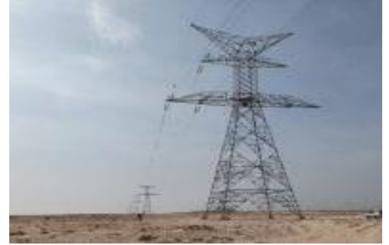
500 kV 256 Km Transmission Line in Egypt
