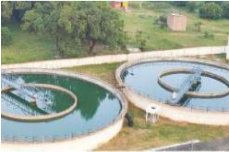
Multi-Villages 30.50 MLD capacity surface water supply scheme | Total length - 792 kms, Bihar
