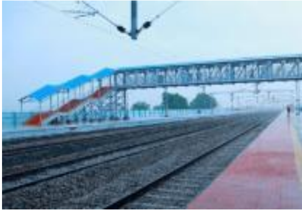
Umdanagar-Mahbubnagar Doubling (Telangana)
