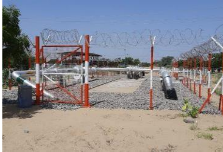
Mangla Intrafield Pipeline Project – Vedanta - Rajasthan
