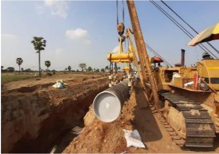
Ennor – Trichy Pipeline Project – IOCL – Tamil Nadu
