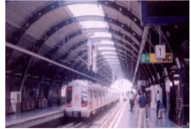
Delhi Metro - Completed Elevated Station
